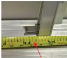
5a: Guide rail measuring. In this example, the guide rails will be 34 5/8" (34 1/2" + 1/8")
