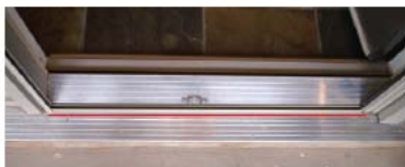
4b: Jamb clip & housing clip on same parallel line
